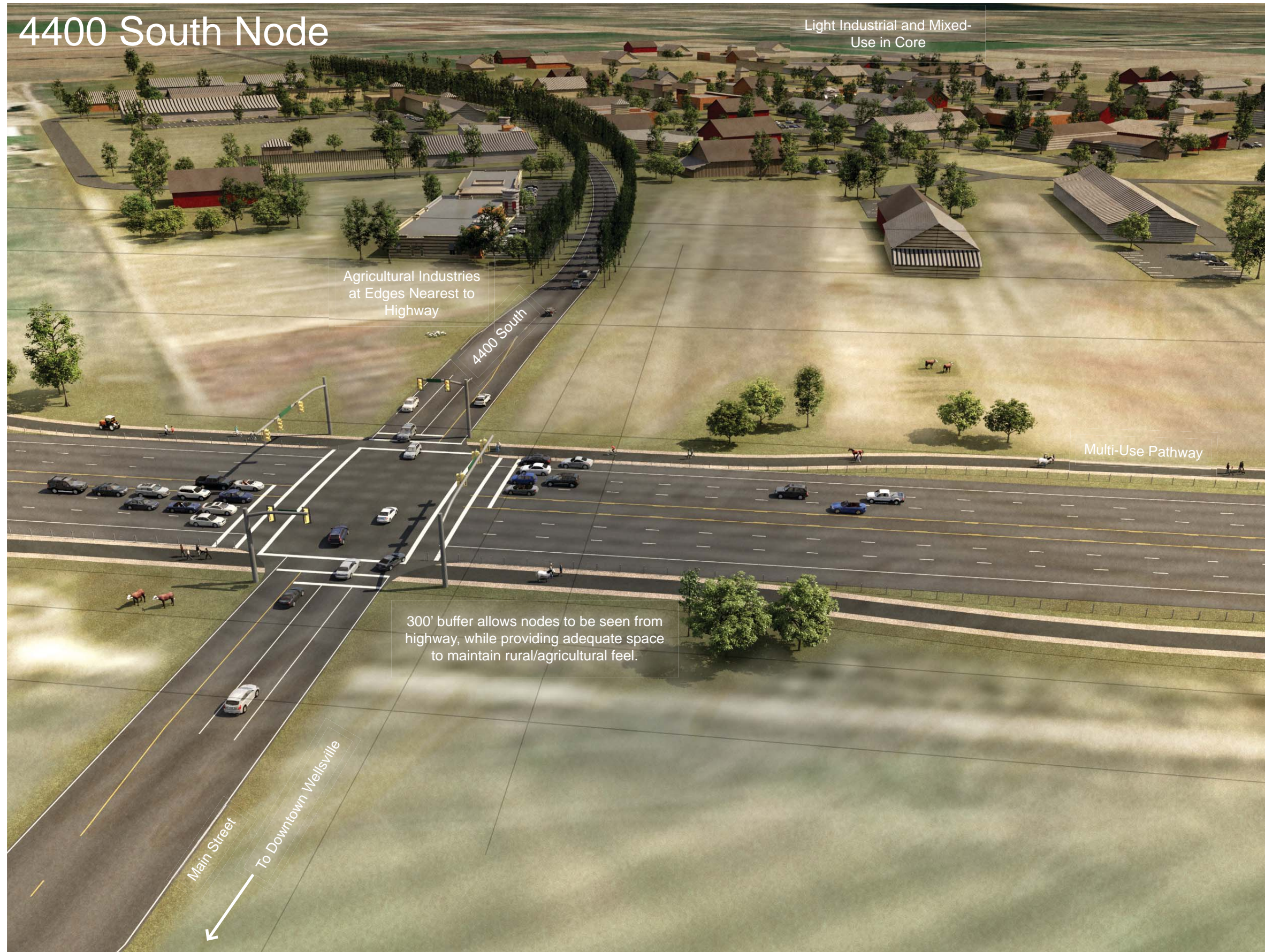
Figure 2-5 Elevated View of 4400 South, Looking East from Intersection.
